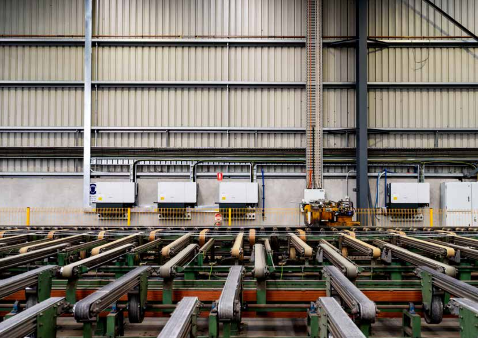
520kW PV Plant Truganina, VIC Australia 🇦🇺
